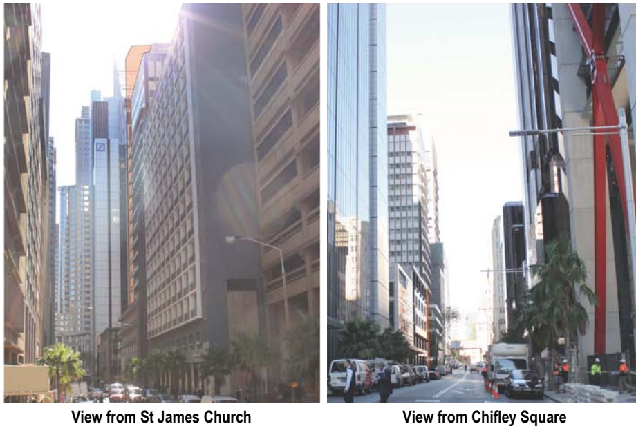
Figure 57 – Views of building envelope in existing built form Source: Hassell
