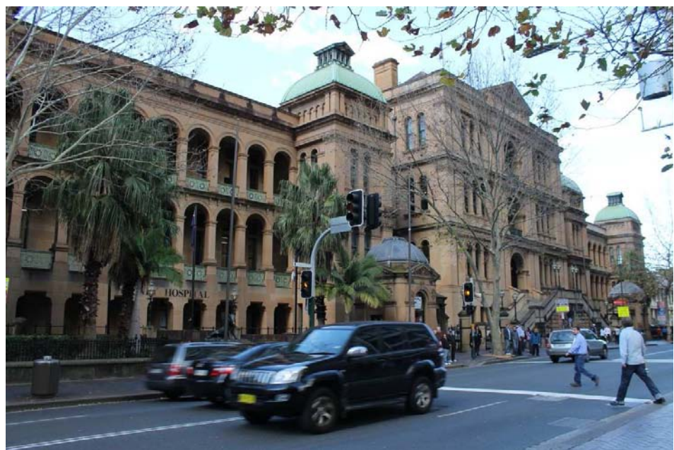
Sydney Hospital group of buildings
